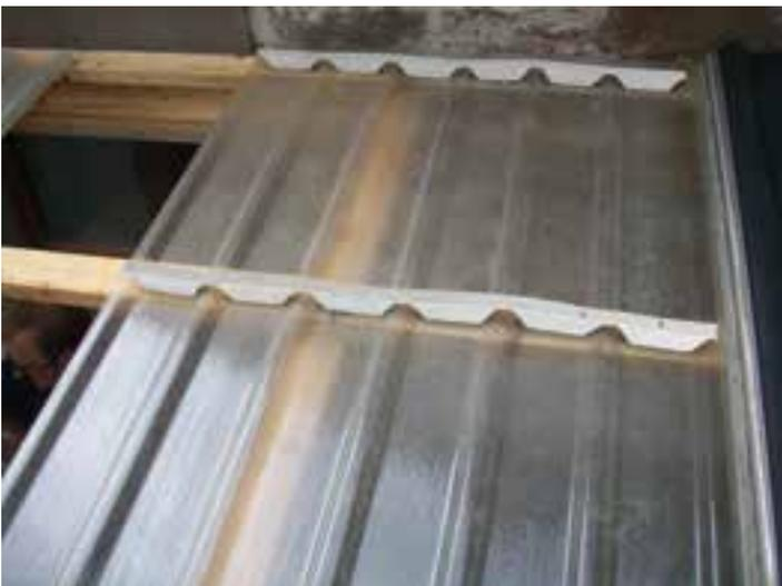
• Low level (17mm) underliner rooflight has been tacked onto timber purlin. Planwell's (white coloured) underliner foam fillers are then placed on top of underliner rooflight then tacked/fix into the timber purlin
