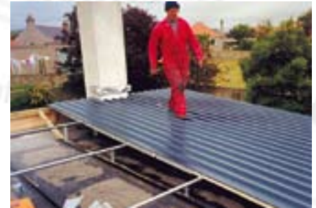
PERMAROOF - strong enough to be walked on
