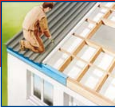
DURING - NEW ROOF BEING FITTED WITH INSULATION
