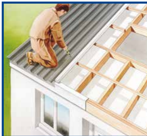
DURING - NEW ROOF BEING FITTED
